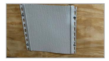
**4)** Fasten a full-length board and batten panel into the nailing flange portion that is holding the cut edge as well. When this is complete you should be able to work in both the left- and right-hand directions.
